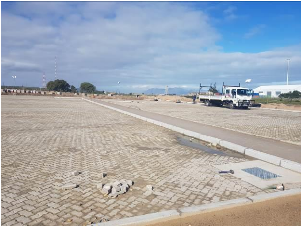
Image 10: Completed paved parking area
