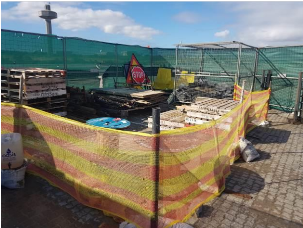
Image 4: Demarcated waste storage area within the site camp
