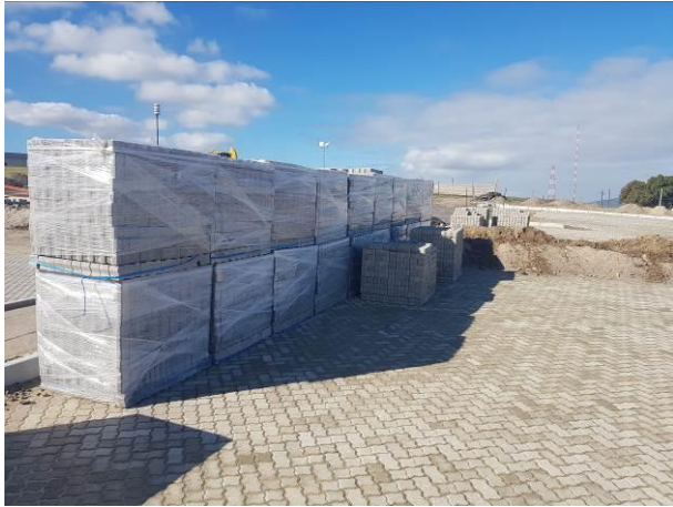
Image 13: Materials stored on site
