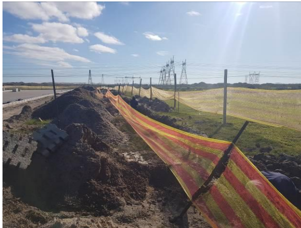
Image 11: Demarcation along excavated trench
