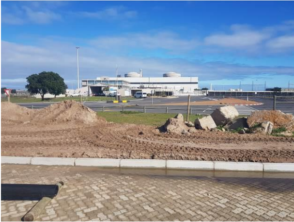
Image 7: Temporary entrance point constructed
