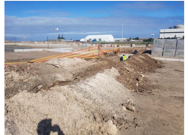
Image 12: Excavated trench and adjacent topsoil stockpiles
